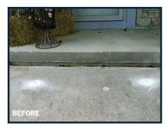
1<sup>1</sup>/<sub>2</sub>-inch to 2-inch holes for cement slurries or traditional mudjacking methods. **ProRise** is lightweight, yet strong and durable, adding minimal weight to the existing soils. Typical densities, or pounds-per-cubic-foot (PCF) weights range from 2.1 PCF up to 4.0 PCF. Strength values range from 38 PSI to 100 PSI. Much higher densities and strength systems are available.
